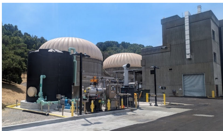
Completed Liquid Organic Waste Receiving Facility
