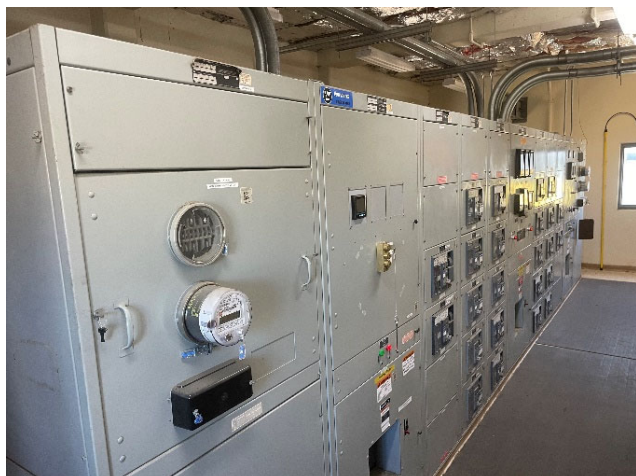
Main switchgear.
