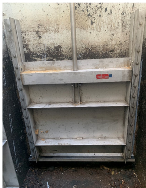
Recently installed stainless steel sluice gate
